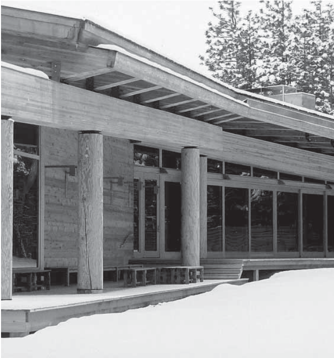
Glulam beams allowed Caldera Hearth Center project designers in Sisters, Oregon to construct an indoor/outdoor roof that added 13,000 square feet of covered space.
