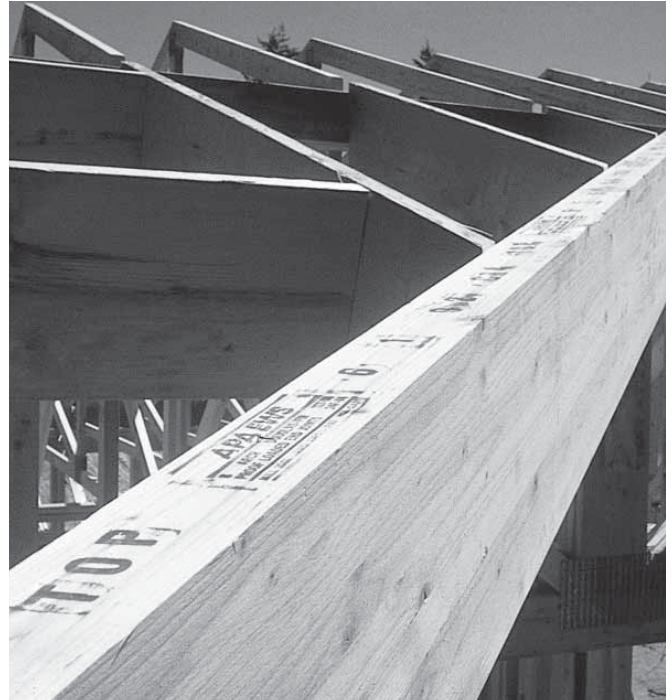
Glulam is manufactured as balanced or unbalanced. Unbalanced beams have different bending stresses in the outer laminations and are clearly marked "top" to ensure proper installation.
